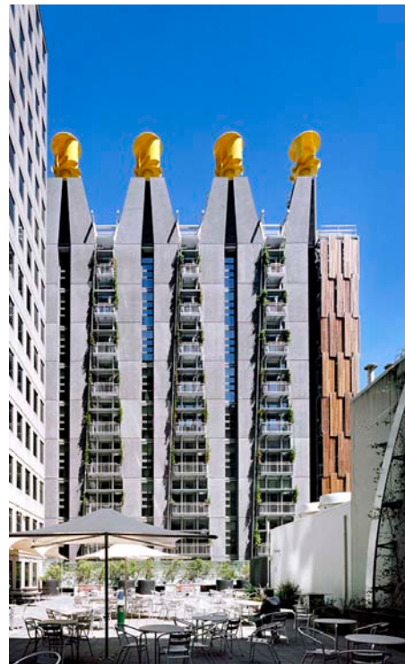
North façade with wind extractors for hybrid ventilation and larger glazing in the lower parts of the building (optimisation)
