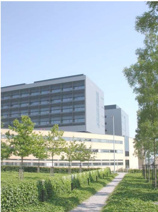
Medical House, Aalborg, Denmark
