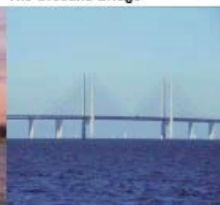
The Öresund Bridge
