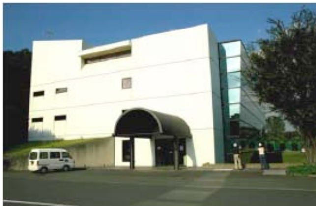
The super energy building at Obayashi TRI
